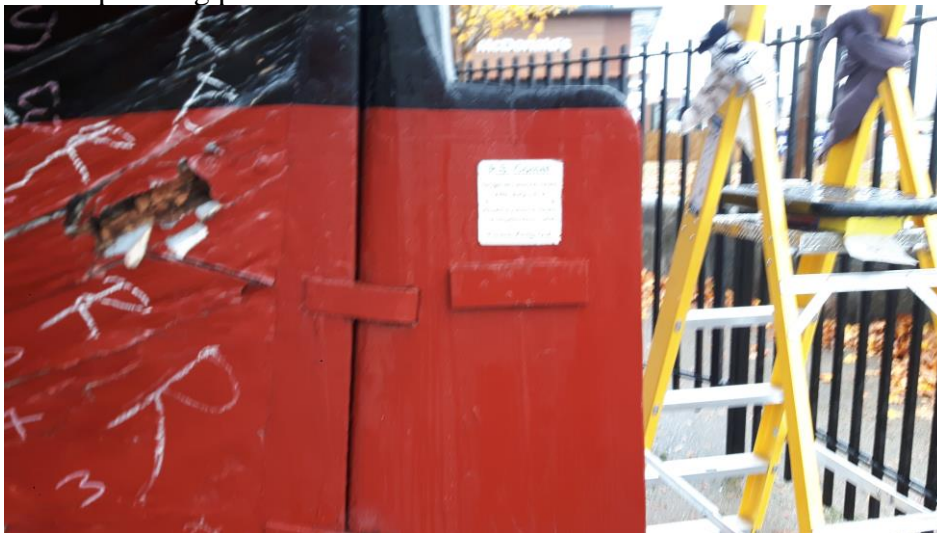
Rotten planking starboard side
